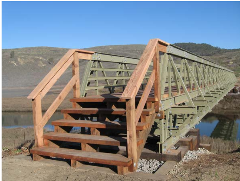
Photo 17.9 - Cutout Stringer Stairway
