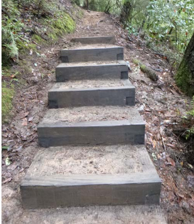
Photo 17.6 - Double Interlocking Steps
