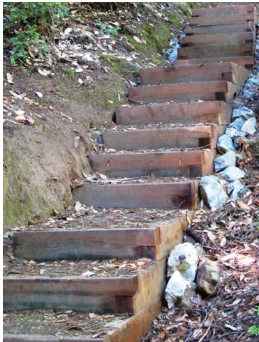
Photo 17.5 - Single Interlocking Steps
