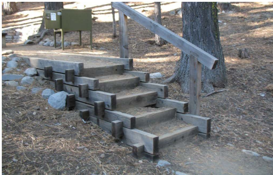
Photo 17.7 - Wooden Cribbed Steps
